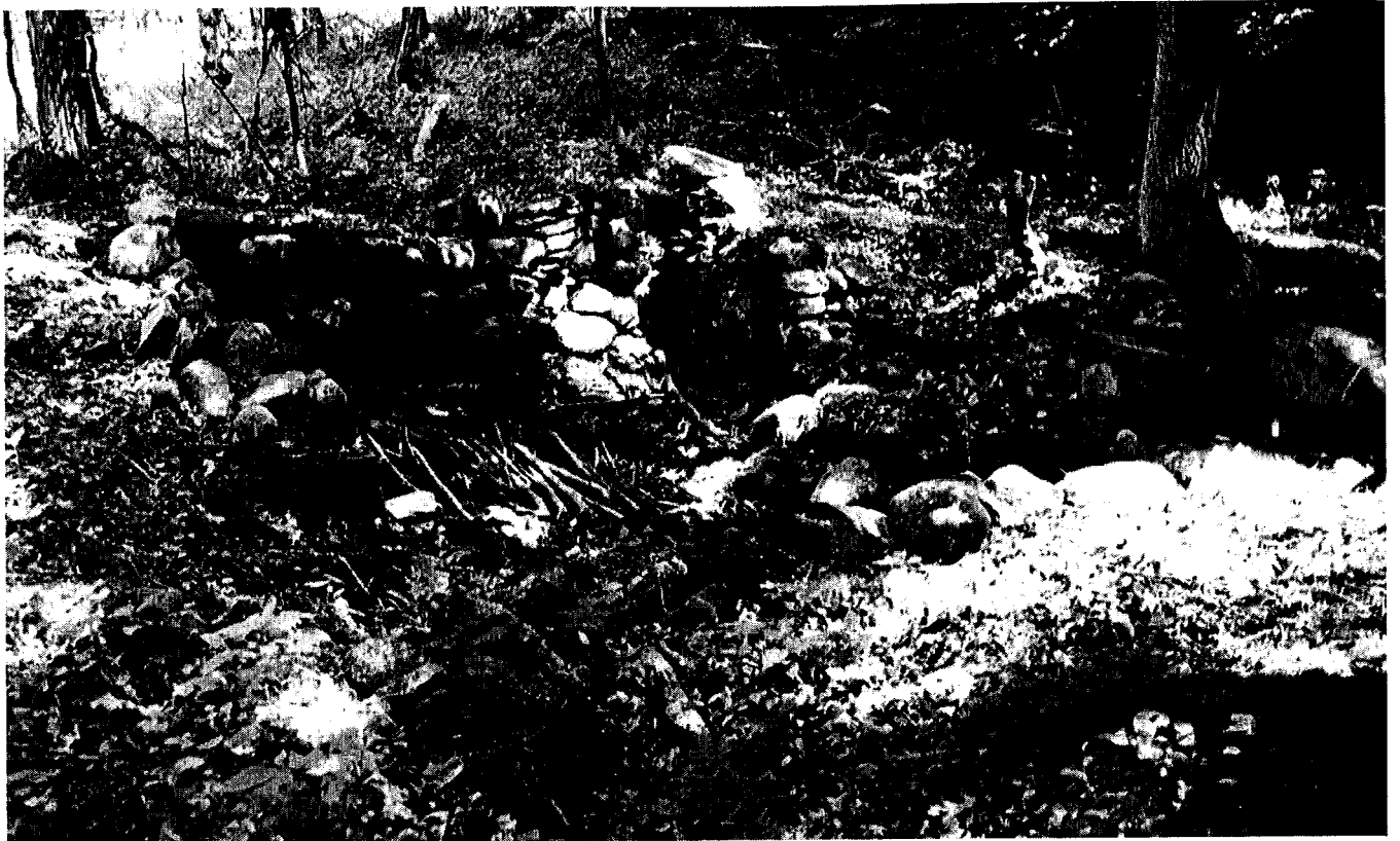
Figure 15. Amos Dixson House foundation, view looking north.
