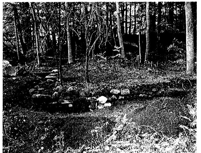
Figure 19. Grove Mather House foundation, view looking north.
