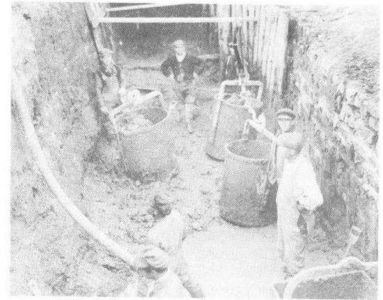
"Laying pipe in the Conduit of the Rochester Water Works"
